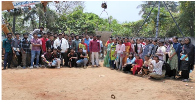
Photograph of students during their visit to the pile foundation construction site
